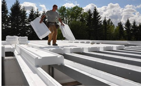
METAL BEAMS & EPS PANELS
